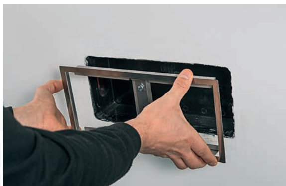
The mounting frame is inserted in the air outlet.
