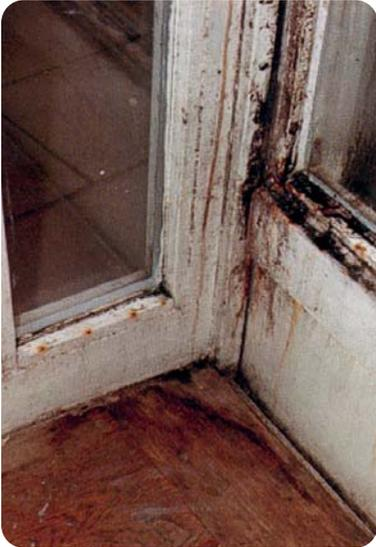
Flats quickly lose their value once mould has settled. The building fabric is permanently damaged and can be remediated only at great difficulty or not at all.
